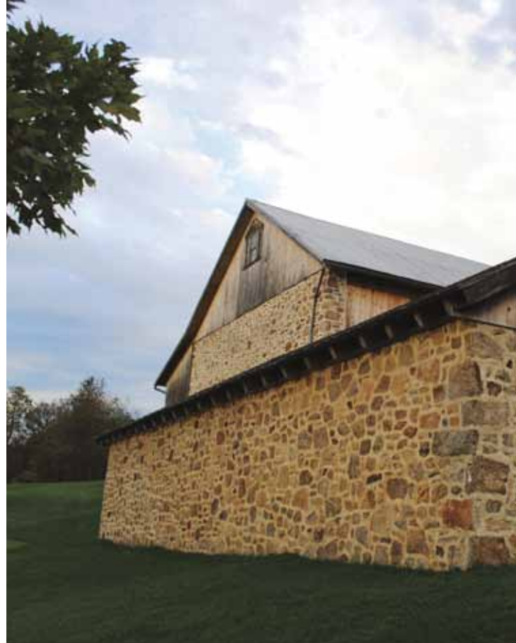
ABOVE, THE RESTORED BARN ACCOMMODATES CASUAL EVENTS. AT LEFT, THE PAR THREE NINTH HOLE, WHICH IS LISTED BY TOM DOAK AS ONE OF THE BEST PAR THREE'S HE HAS DESIGNED.
